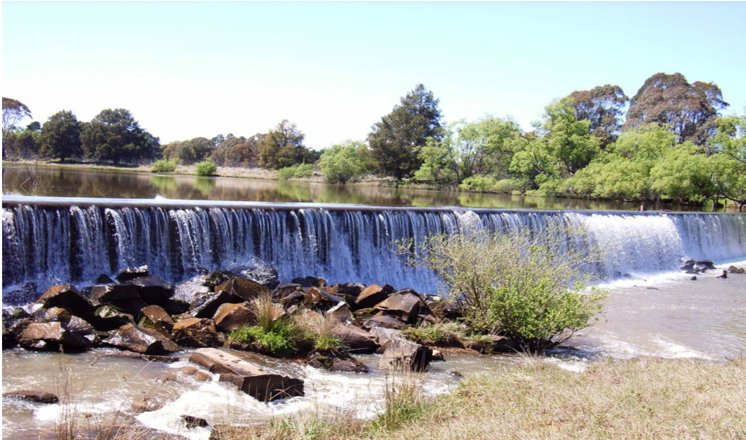
Wingecarribee River Weir
